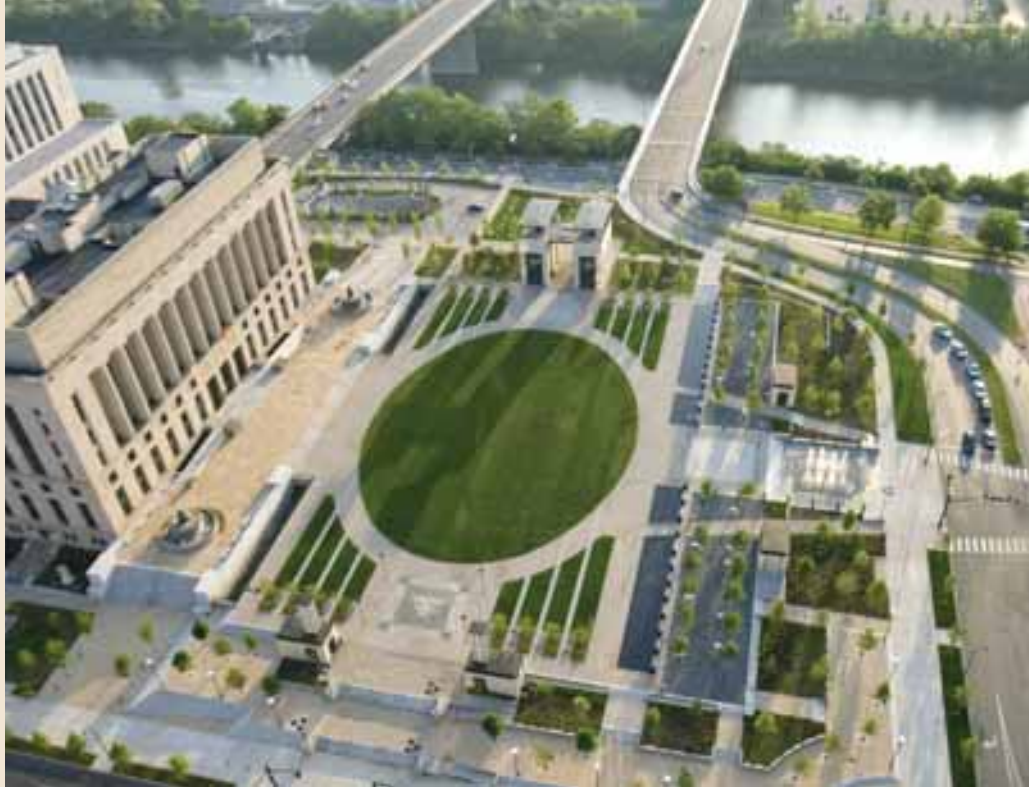
Nashville's source of drinking water, the Cumberland River, runs 120-feet away from the site. Mitigating the effect of stormwater runoff on the Cumberland was a significant concern in the design. (Photographer: Bob Schatz)
